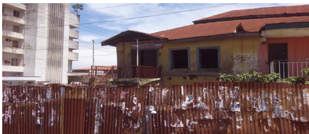
Figure 9: A building about to be converted from residential to commercial use along Adesida / Oyemekun road, Akure.
