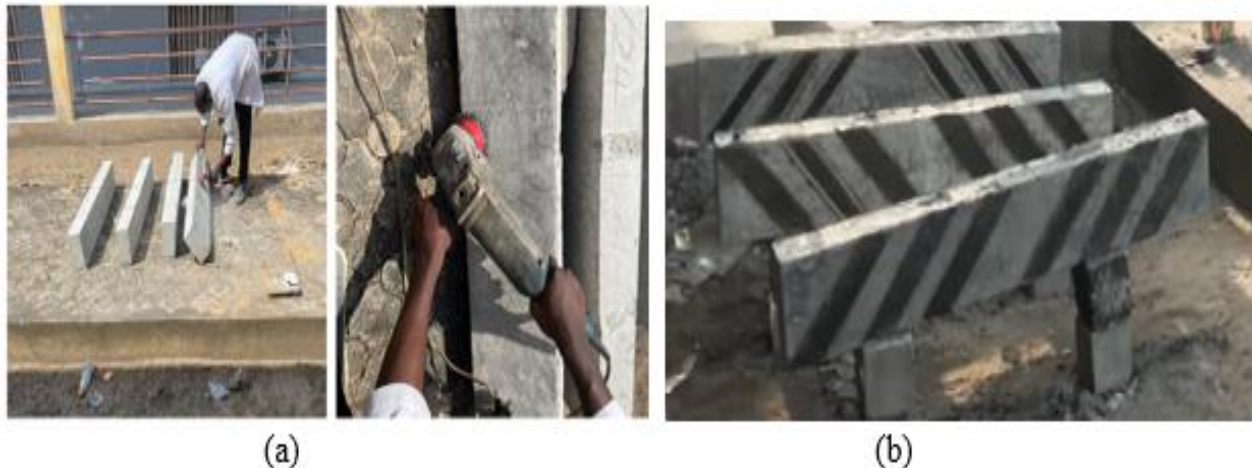
Plate 2: (a) Application of Concrete (b) Surface preparation
