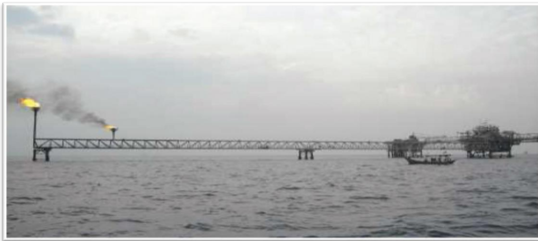
Figure 6: Offshore oil and gas platform (Source: Heri, et al, 2018)
