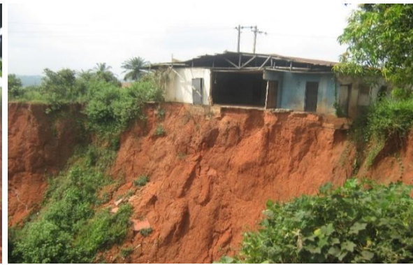
Plate 8: One of the residential buildings in Ogbeson quarters being threatened by Queen Ede erosion
