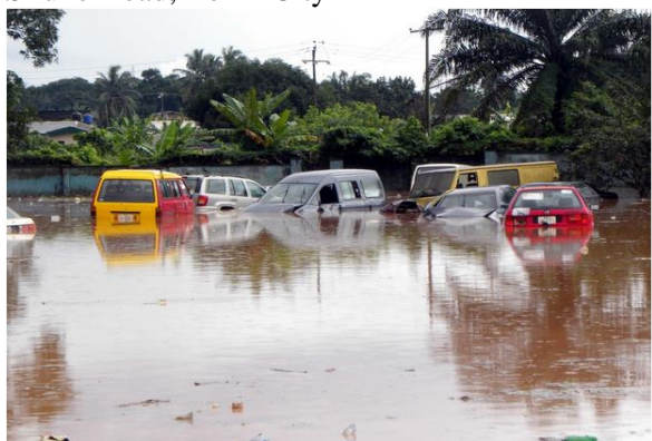
Plate 3: Flooding of Ugbowo/Oluku quarters, Benin City
