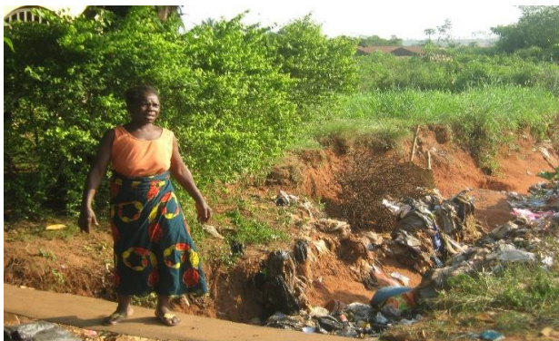
Plate 9: Road completely cut-off by erosion in Ogbeson quarter Benin City
